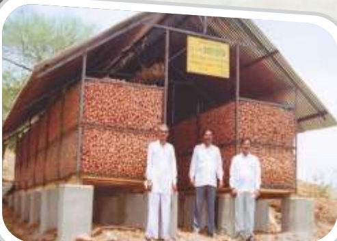
Onion Storage Structure
